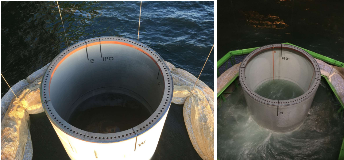
Figure 2: Top view of previous project HSD system deployed around a pile (left: net being deployed with ballast box underwater, right: net being retrieved in the ballast box)
